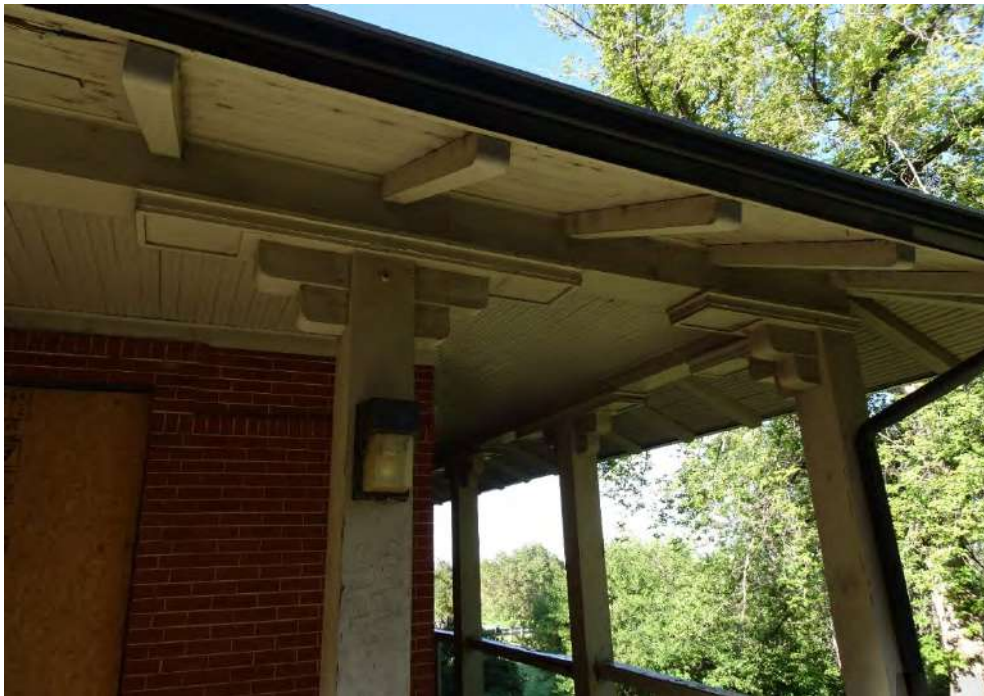
Priest's House rounded porch brackets and rafters details, facing north-northeast.
