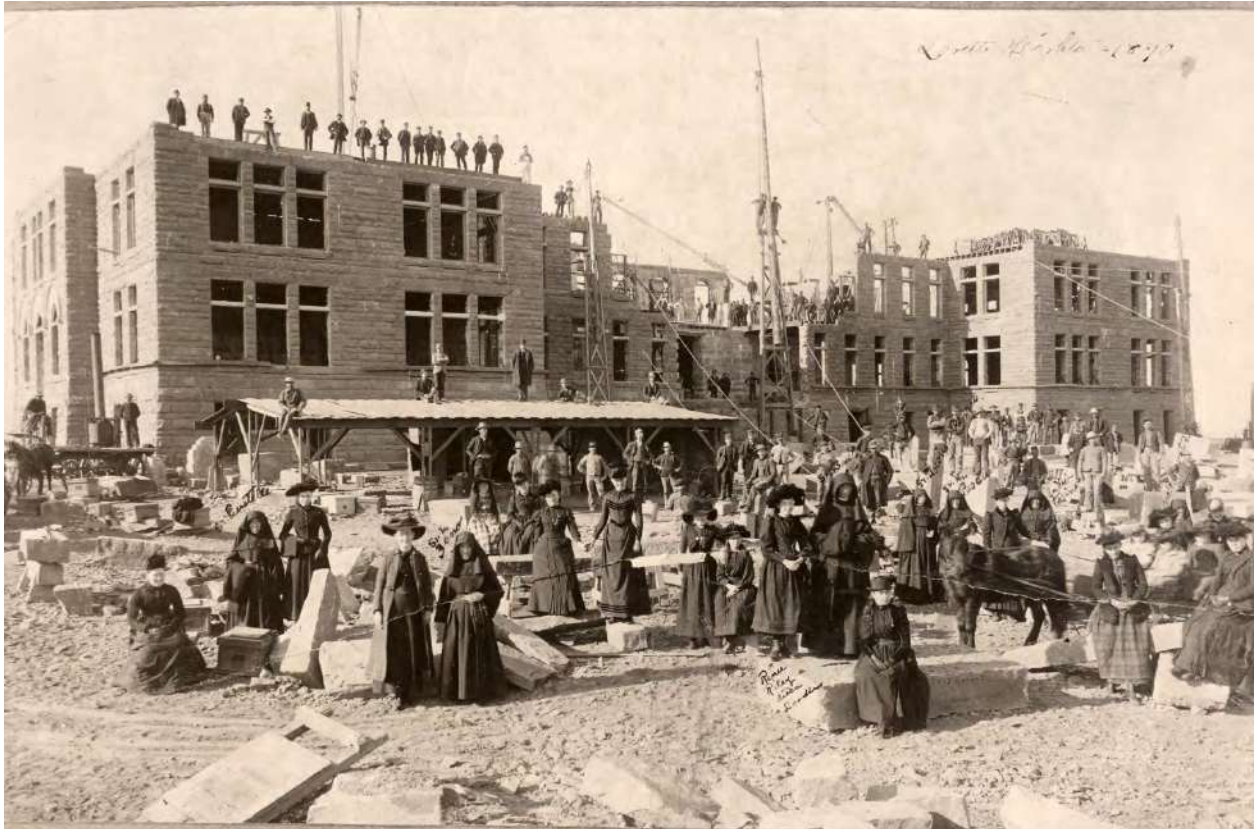
Loretto Heights Academy's Administration Building, camera facing northwest, under construction in 1891, witnessed by Loretto Sisters, workers, and others. The red sandstone came from a quarry in Manitou Springs, brought by railroad to within a mile of Mt. Loretto. See the completion photo on the front cover of this report. Regis Archives.
