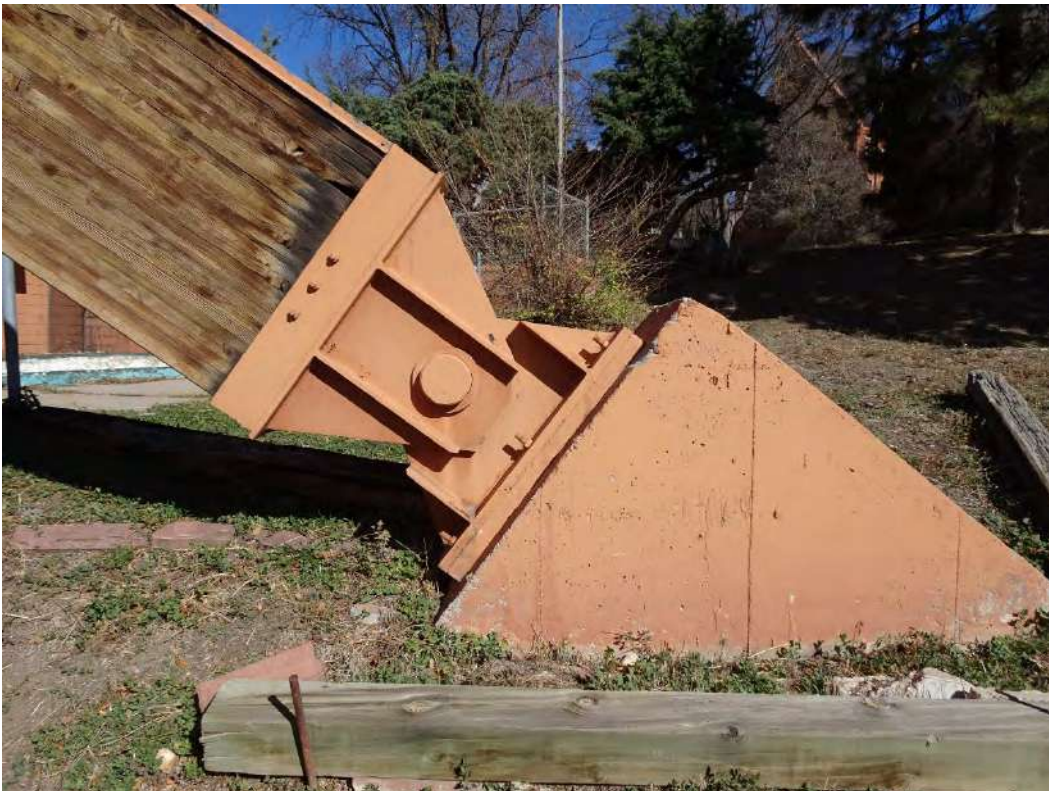
Swimming Pool detail of east-corner laminated-beam hinge and concrete anchor, facing northeast.
